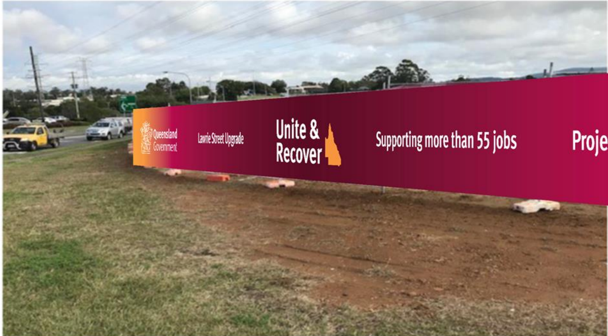
Figure 13.1 – Example of mesh screening
