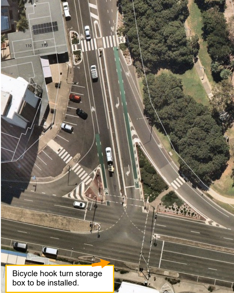
Figure 4 Sixth Avenue improved pedestrian crossing, bike lanes and protected right turn for bike riders (Source: Nearmap 2020)
