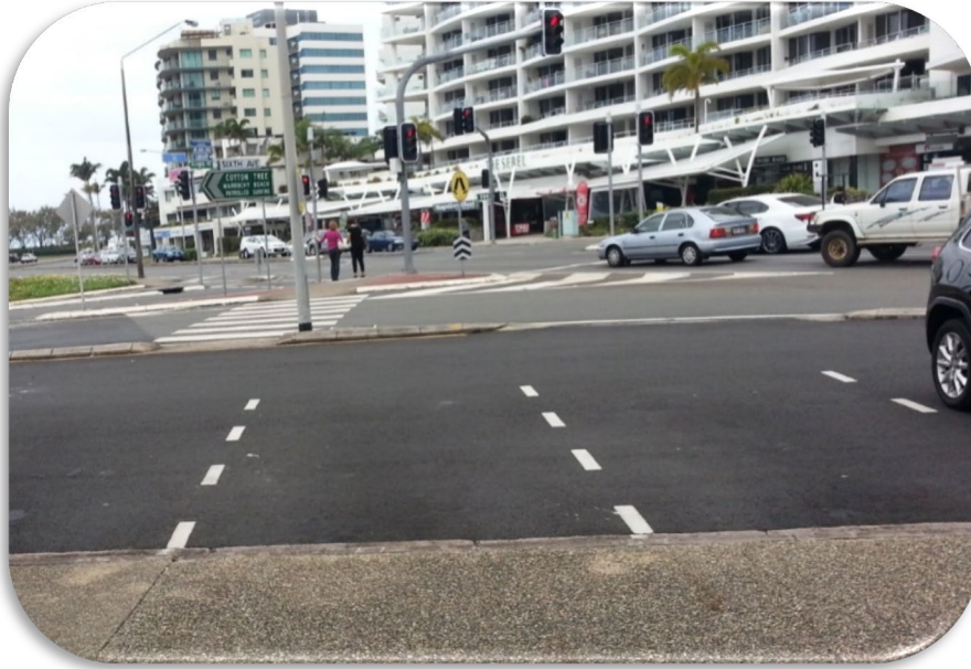
Figure 3 Existing car parking provision off Sixth Avenue Aerodrome Road, Maroochydore, 2015
